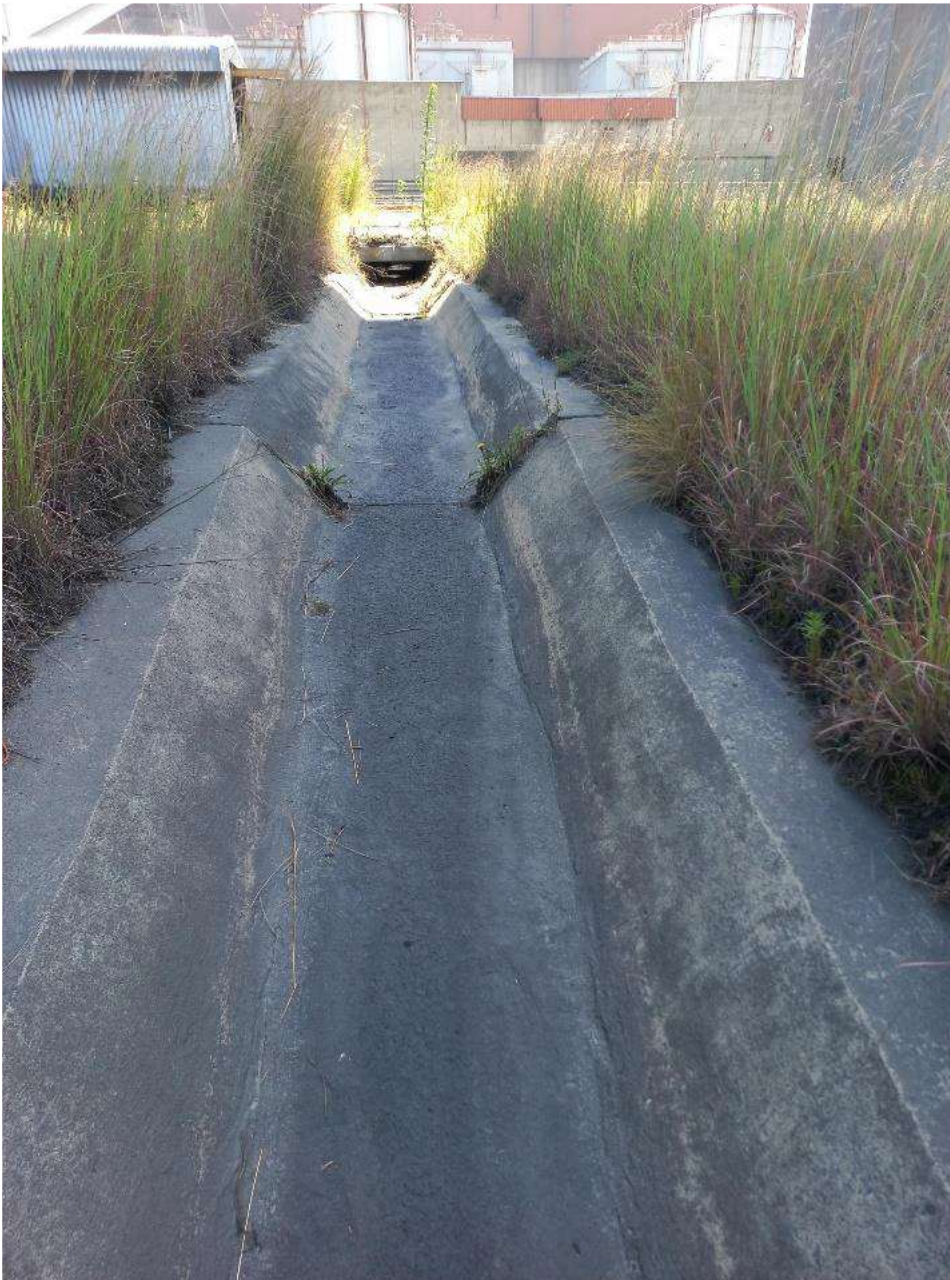
Figure 24: Concrete V-Drains from Silt Traps to Coal & Ash Settling Ponds
