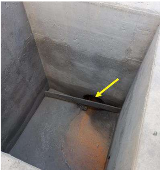
Figure 5: Outlet Pipe to Station Drains
