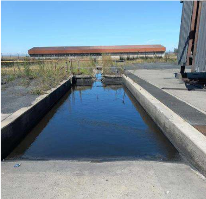
Figure 23: Silt Trap at Each Silo
